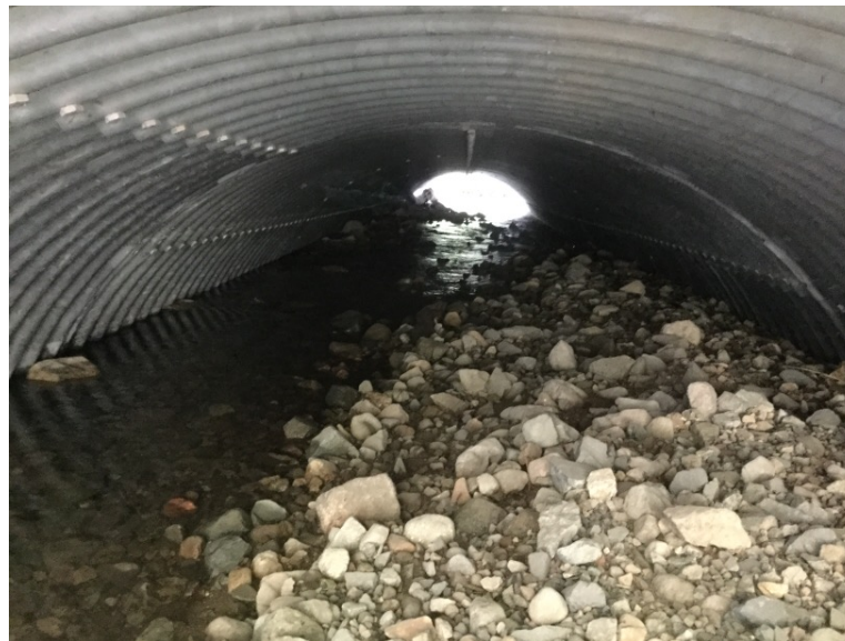
Looking through culvert from inlet
